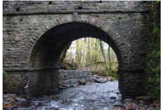
Bridge over Nant Clydach © Jenny Lunn
